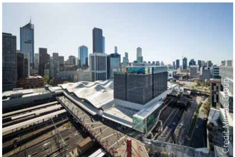
Top: King's Cross station in London redeveloped. Above: Mirvac's AGL building in Melbourne close to major transport hub, Oculus.
