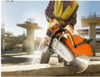
Above: Cut-off saw with water suppression
