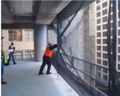
Figure 1: Debris perimeter protection
