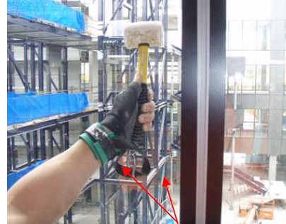
Figure 2: Hand tool secured to wrist by a lanyard
