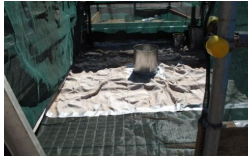
Figure 8: Screen on scaffolding
