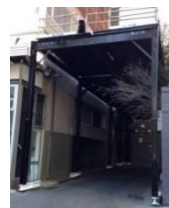
Figure 9: Overhead protective structure – Type B Hoarding
