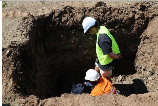
Figure 8: Backfill. Geofab used as marker layer at approximately 600mm below surface
