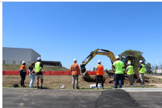
Figure 8: Backfill. Geofab used as marker layer at approximately 600mm below surface
