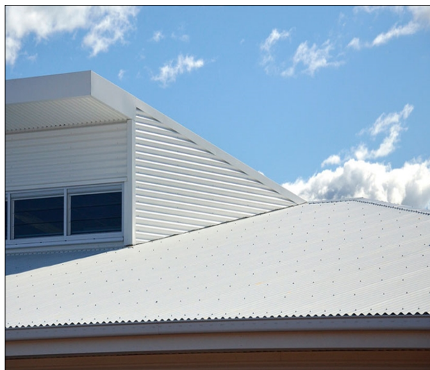
Figure 8 - Illustration of a light coloured (reflective) roof sheeting.
