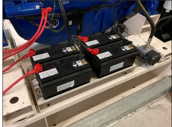
Photo 2 Battery storage in North Tower, level B1, Diesel Generator Room.
