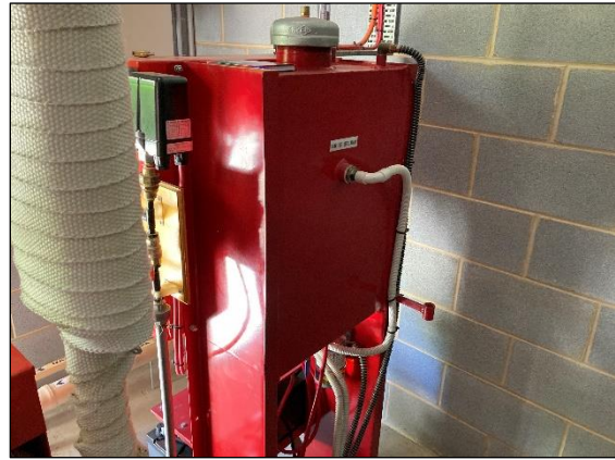
Photo 8 Diesel fuel storage in North Tower, Level 1, Sprinkler Pump Room.
