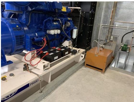
Photo 3 Diesel Fuel Storage (Brake Tank) in North Tower, level B1, Diesel Generator Room.
