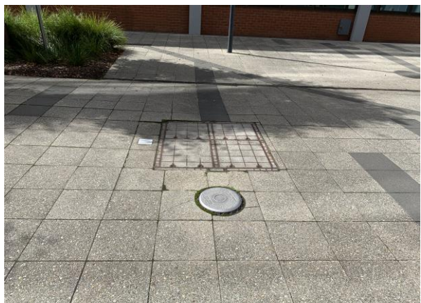
Photo 6 Underground diesel fuel storage tank, North Tower, Level 1 (exterior), adjacent loading dock entry.
