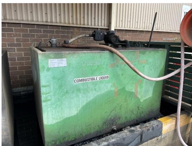
Photo 23. Building 1, East side, north area, diesel tank – fuel tank.
