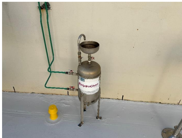
Photo 10. Unlabelled dosing pot on Level 32 roof.
