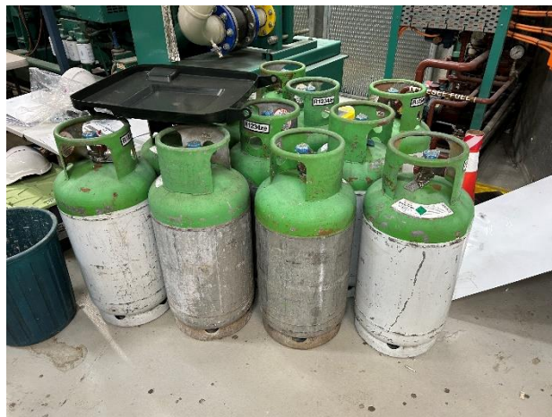
Photo 08. Unsecured refrigerant cylinders in Generator Room.
