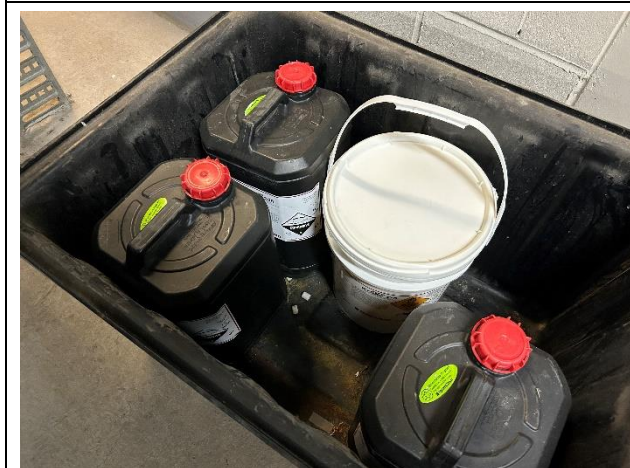
Photo 05. Incompatible hazardous chemicals stored together in Level 32 Boiler Room.
