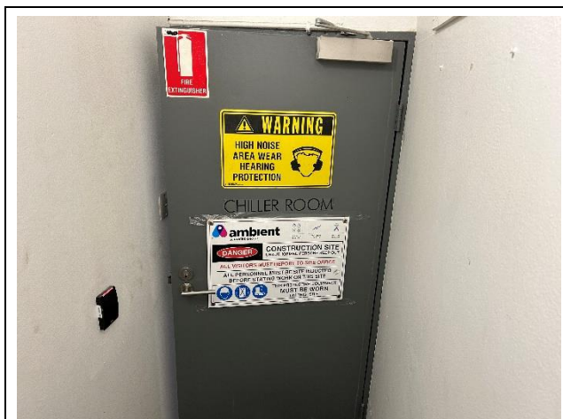
Photo 01. No Class 2.2 placard at entrance to Chiller Room.
