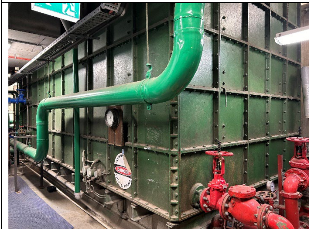
Photo 15. 10 Bond Street, Cooling Tower Plant Room, hydrant tank
