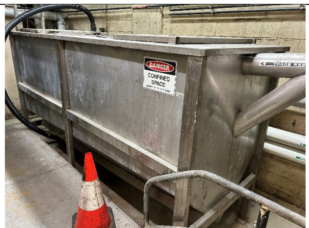
Photo 12. 20 Bond Street, Grease Trap Room, grease trap
