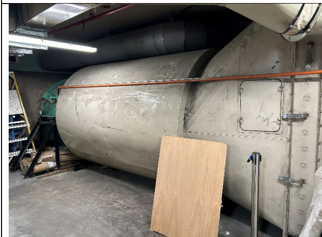
Photo 17. 10 Bond Street, Level B4, plant room adjacent 10 Bond St lifts, smoke exhaust fan chamber
