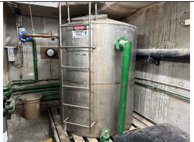
Photo 16. 10 Bond Street, Cooling Tower Plant Room, flusherette tank
