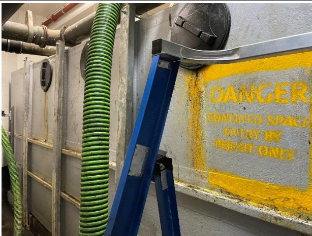
Photo 11. Level B2, Grease Arrestor Room, adjacent parking space 100 – grease trap.
