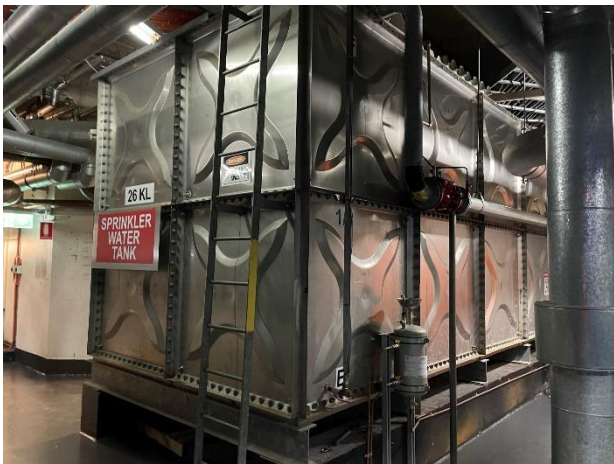
Photo 03. Level 8, Level Chiller Room (sprinkler system) – water tank.
