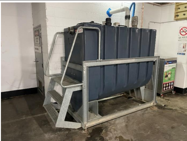
Photo 05. Level B6, Loading Dock, adjacent Grease Arrestor Room – grease trap.
