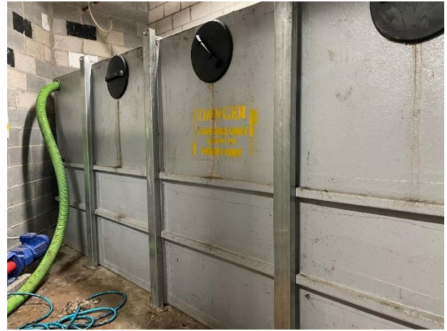
Photo 10. Level B2, Grease Arrestor Room, adjacent parking space 102 – grease trap.
