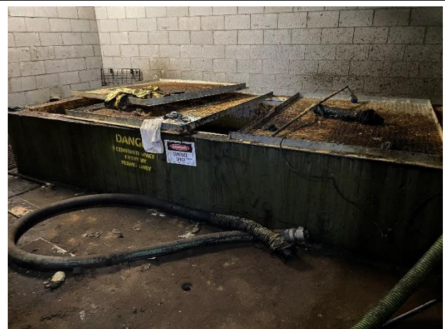
Photo 12. Level B2, Grease Arrestor Room, adjacent parking space 109 – grease trap.
