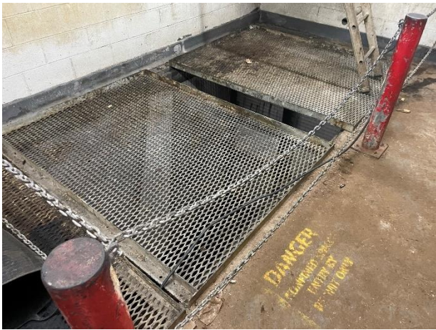
Photo 07. Level B3, Greenwood Plaza Loading Dock, Grease Arrestor Room – grease trap.
