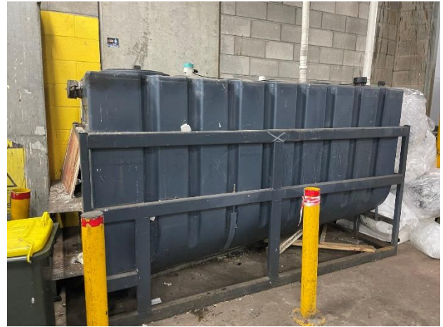
Photo 08. Level B3, Greenwood Plaza Loading Dock – grease trap.
