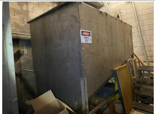
Photo 06. Level B6, Grease Arrestor Room – grease trap.
