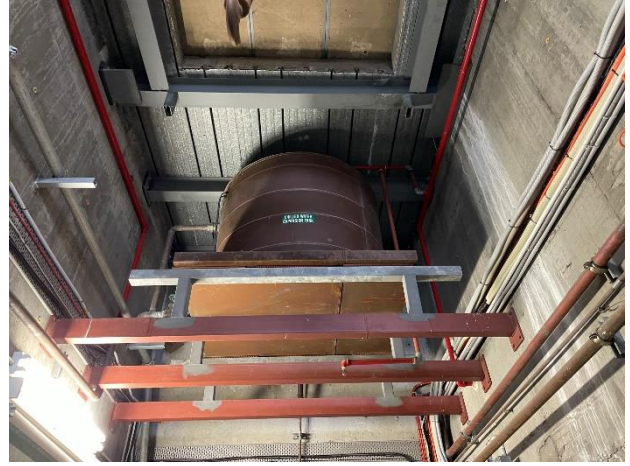
Photo 02. Level 35, Cooling Tower Plant Room, high level, above entrance to Hydrant Pump Room (chilled water expansion tank) – water tank.
