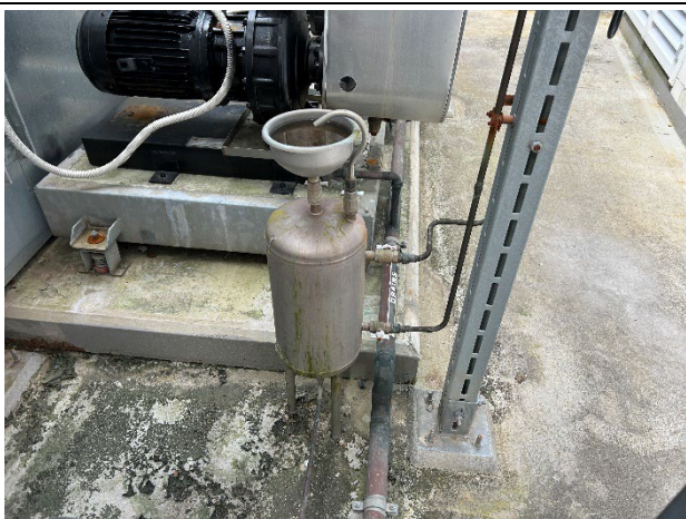
Photo 07. Unlabelled chemical container in Dalley Street Level 4 Cooling Tower Area.
