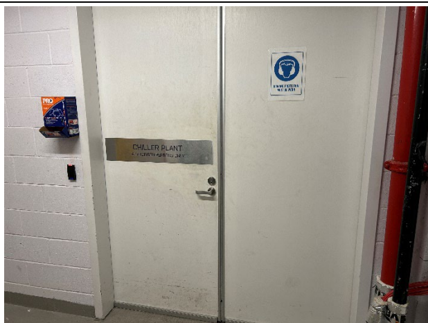
Photo 01. No Class 2.2 location placard at entrance to Dalley Street Level 3 Plant Room.
