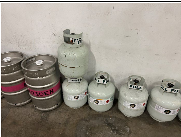
Photo 11. LPG cylinders in Level US Loading Dock not appropriately secured.
