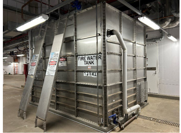
Photo 08. Level 1, Dalley Street, Water Tank Room – fire water tank.
