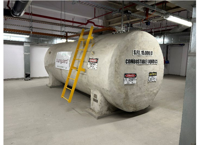
Photo 10. Basement Level, Dalley Street, Diesel Tank Room – large diesel tank.
