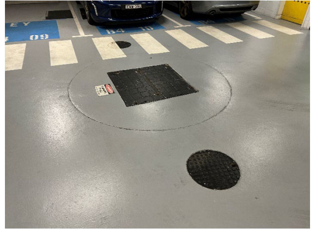
Photo 14. Level B4, carpark, adjacent parking space 10 – grease trap.
