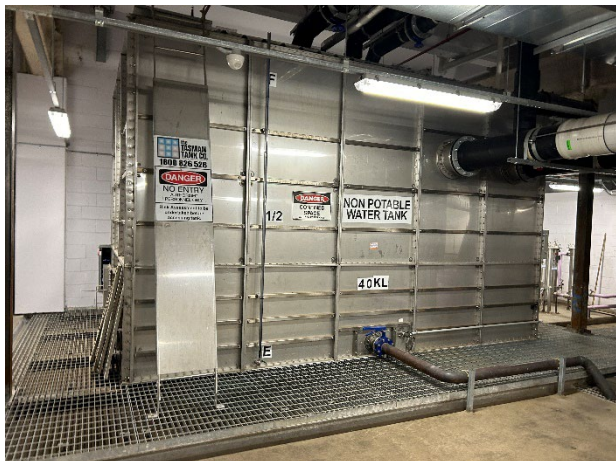
Photo 05. Level 1, Dalley Street, Water Tank Room – non-potable water tank (E).
