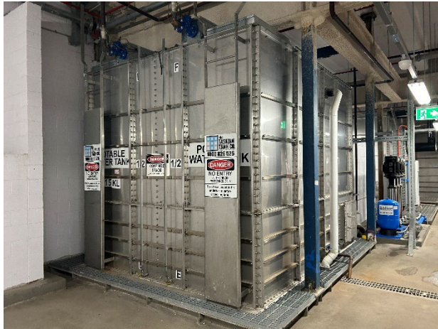
Photo 07. Level 1, Dalley Street, Water Tank Room – potable water tank.
