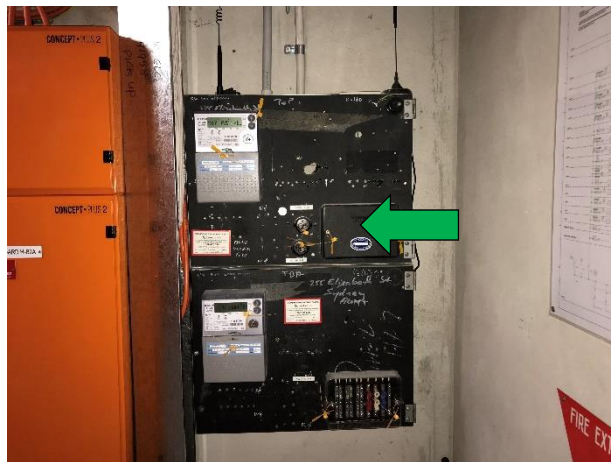
Photograph 8: Level B2, main switch room, electrical backing board – non-asbestos containing bituminous backing board.
