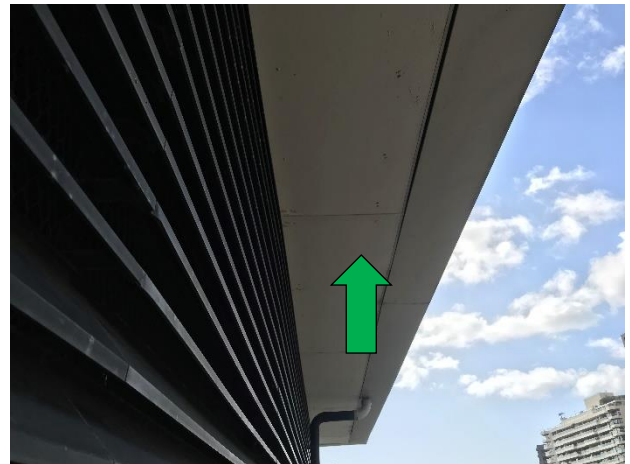
Photograph 4: Level 17, exterior, perimeter, eaves – non-asbestos containing fibre cement sheeting.
