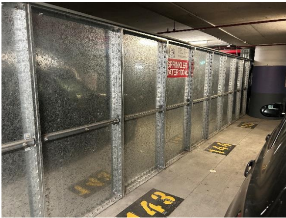
Photo 09. Level B6, parking bays 141-145, sprinkler water tank.
