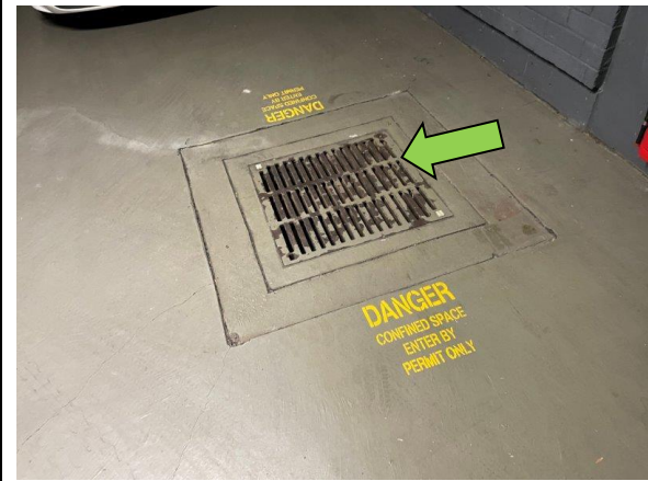
Stormwater / sump with appropriate confined spaces warning signage
