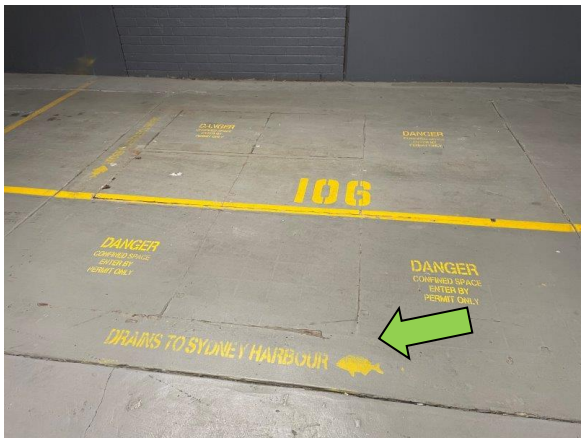
Sub Soil Access Pits with appropriate confined spaces warning signage
