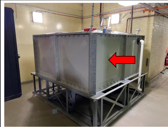
The 4,000L water tank on Level 31 was not labelled as a confined space
