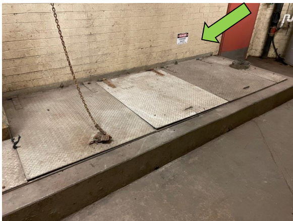
Grease trap with appropriate confined spaces labelling
