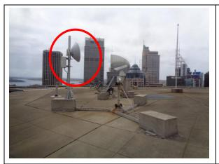
Potential radio frequency radiation equipment recently installed on the roof level
