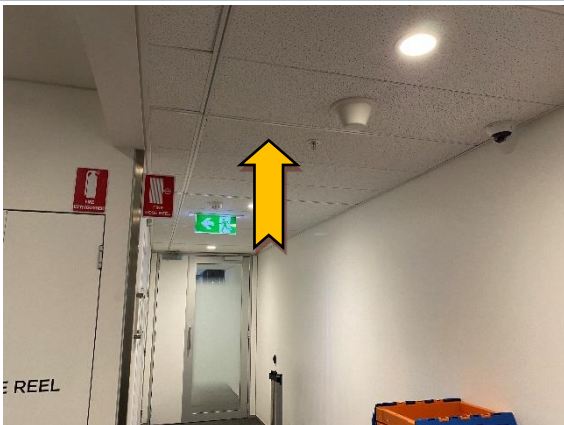
Photo 5 Interior: levels 1 – 32, lift lobby, ceiling – suspected SMF containing compressed ceiling tiles.
