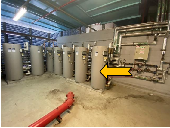
Photo 7 Interior: level 4, plant room, hot water heater – suspected SMF containing internal insulation material.
