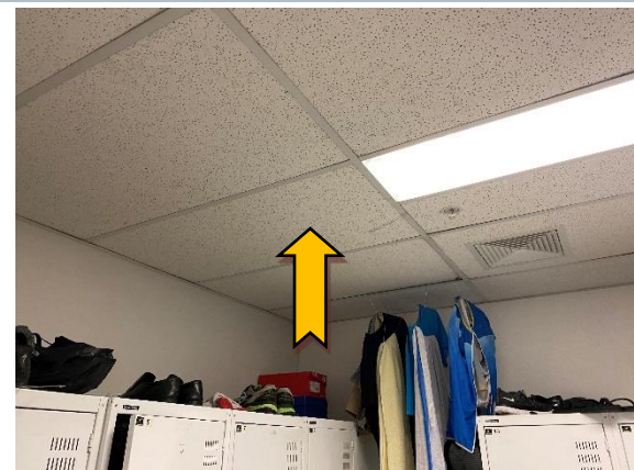
Photo 4 Interior: levels 1 – 32, bathrooms, ceiling – suspected SMF containing compressed ceiling tiles.
