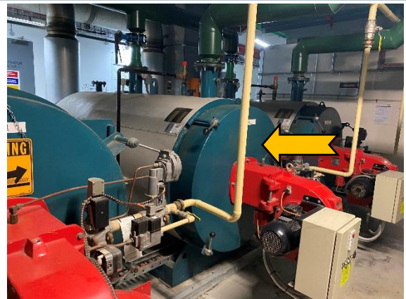
Photo 6 Interior: level 4, plant room, boiler – suspected SMF containing internal insulation material.
