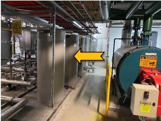
Photo 1 Interior: level 33, plant room, throughout, hot water heater – suspected SMF containing internal insulation material.
