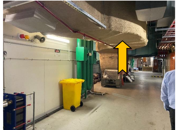
Photo 2 Interior: level 33, plant room, throughout, air conditioning ductwork – suspected SMF containing internal insulation material.
