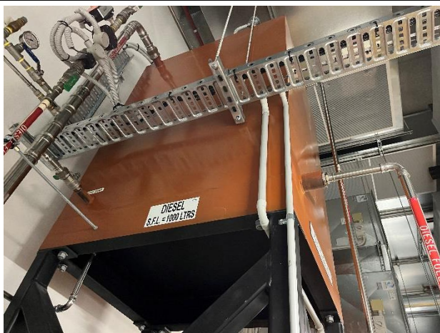
Photo 03. Level 4, Plant Room, WBC Generator Room, Day Tanks A and B – Fuel Tank
