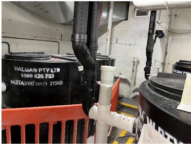
Photo 07. Level P1, Plant Room adjacent Mail Room – Grease Traps x 3
