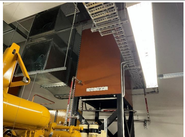
Photo 04. Level 4, Plant Room, WBC Generator Room, Day Tanks A and B – Fuel Tank
