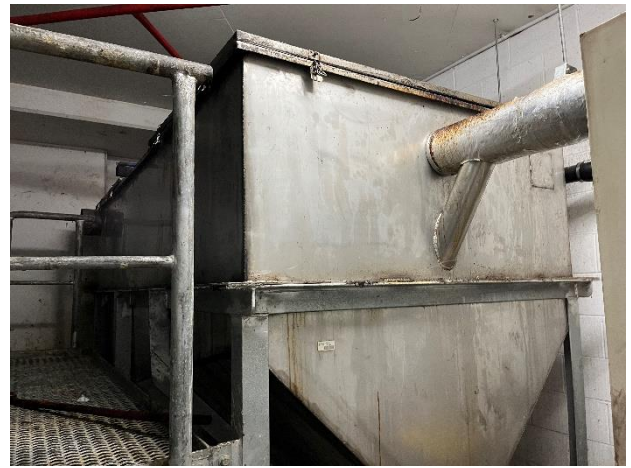
Photo 10. Level P1, Plant Room adjacent parking bay 71 and 41 – Grease Trap
