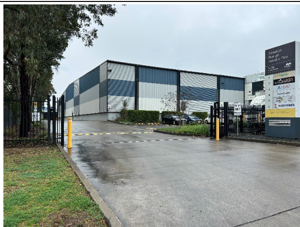
Photo 02. No HAZCHEM outer warning placard at vehicle entrance to site.
