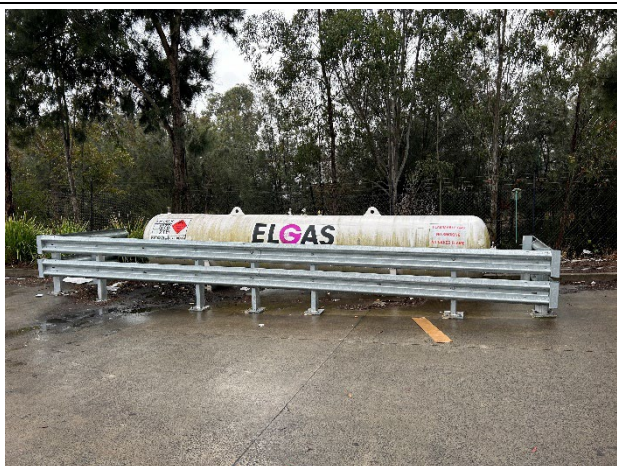
Photo 01. Bulk LPG tank with Class 2.1 location placard.
