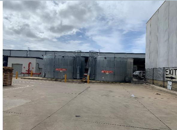
Photo 8 Exterior, ground level, adjacent fire pump room, water storage tank, sprinkler tank (185kL) x 2
