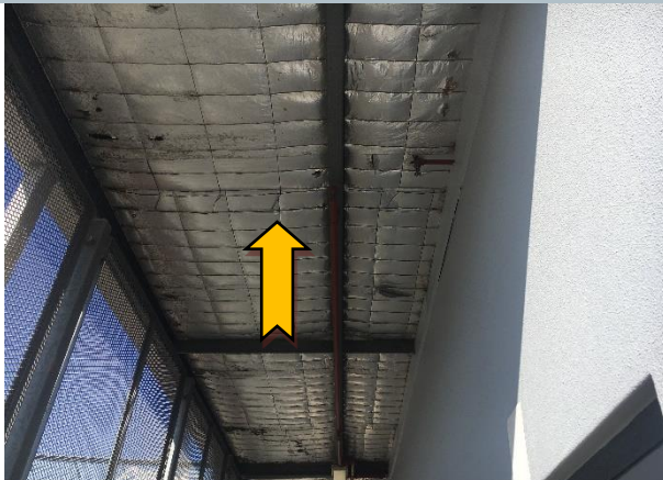
Photo 3 Exterior: substation, eaves – suspected SMF containing insulation.
