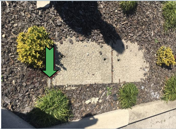
Photo 1 Exterior: carpark in front of office building, adjacent main carpark entrance, pit – non asbestos containing fibre cement pit lining.
