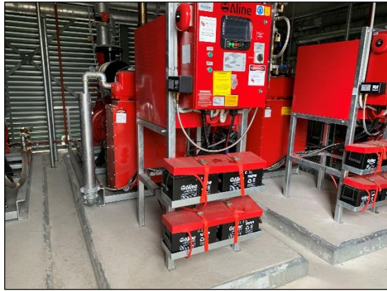
Photo 1 Sprinkler pump room
