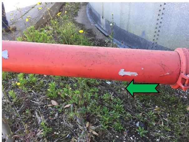
Photo 3 Exterior: throughout, pipework, red paint – non lead containing paint.
