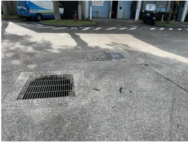
Photo 13. Adjacent units 18, 17 and 5, on road, stormwater drain and unknown pit
