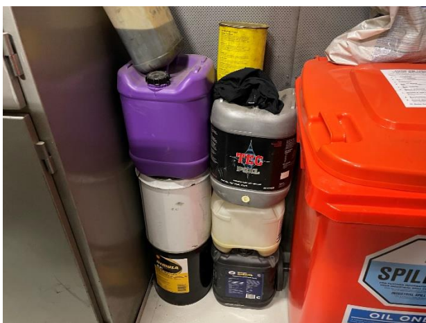
Photo 01. Class 3 and Class 8 chemicals stored together in Generator Room.
