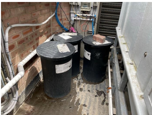
Photo 05. Water treatment chemical storage in Level 7 cooling tower area.
