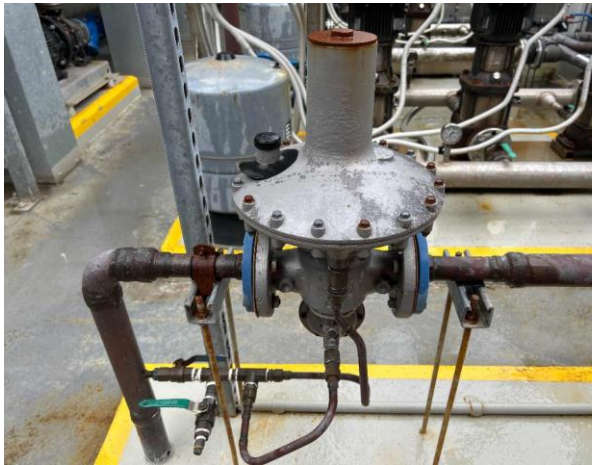
Line ID 1: External, L33, Throughout, Gasket to Gas Supply Valve, Gasket Material - No Asbestos Detected
