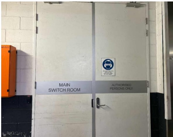
Line ID 20: Internal, B1, Main Switchroom – No Access
