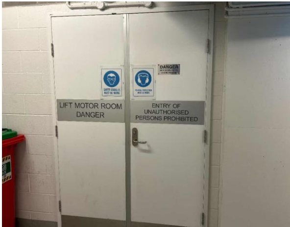
Line ID 22: Internal, L20, Lift Motor Room – No Access
