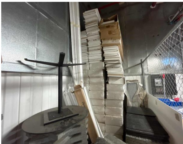
Line ID 14: Internal, L32, Plant Room, Southwest Corner, Storage Cage, Compressed Ceiling Tiles - Suspected SMF
