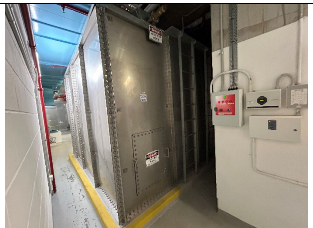
Photo 06. Level 3 Plant Room, hydrant water tank.
