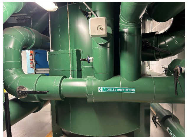
Photo 04. Level 30 Plant Room, chilled water tank.
