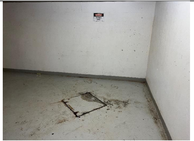
Photo 20. Level B3, Sprinkler Pump Room, unknown pit.
