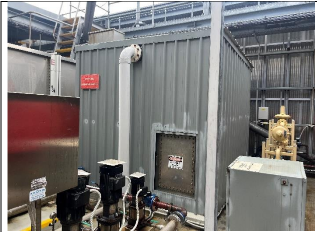
Photo 01. Cooling Tower Area, potable water tank.
