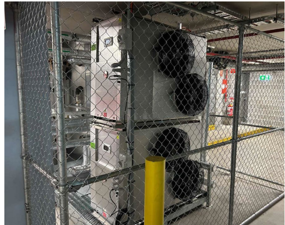
Line ID 28: Internal, B3, Carpark, Caged Area, AC Units, R1234yf - Non ODS Refrigerant
