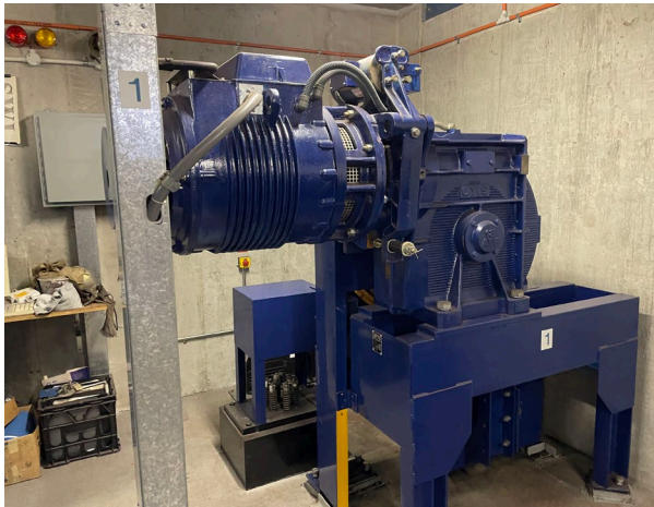
Line ID 1: Internal, L16, Lift Motor Room, 5 x Lift Motors, Friction Pads - No Asbestos Detected
