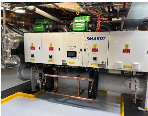
Line ID 29: Internal, L15, Chiller Room, Chillers, R1234ze Refrigerant - Non ODS Refrigerant
