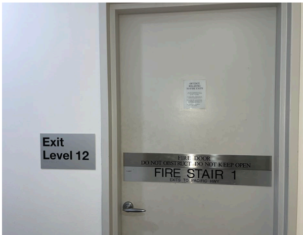
Line ID 2: Internal, All Levels, Stairwells and Plant Rooms, Various Throughout, Fire Door Core - No Asbestos Detected
