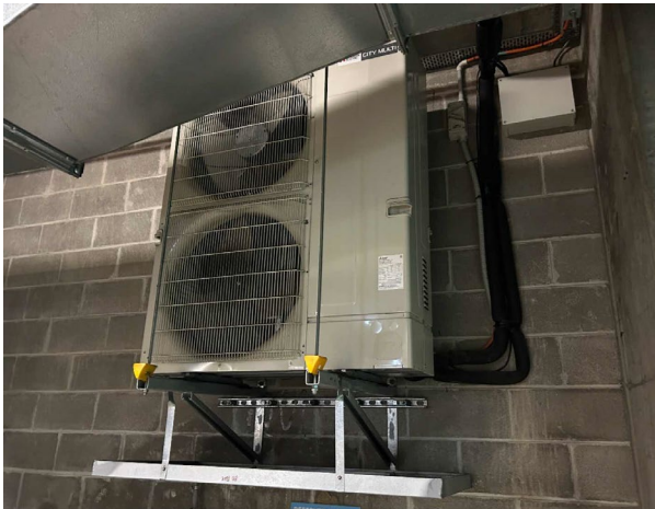
Line ID 27: Internal, B1, Carpark, Parking Space 13, AC Unit, R410A Hydrofluorocarbon (HFC) - Non ODS Refrigerant
