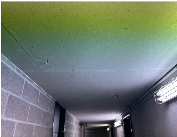
Line ID 8: Internal, L15, Corridors, Ceiling, Insulation Board - No Asbestos Detected
