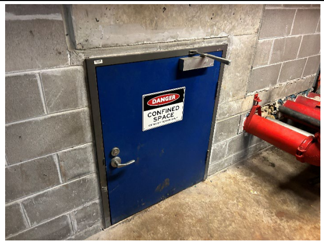
Photo 02. Fire Pump Room – sump pump pit.
