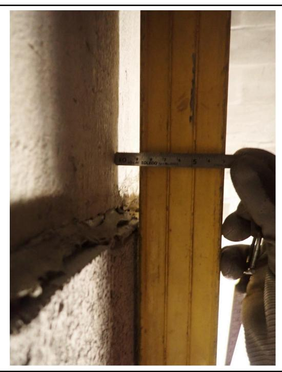
Date: 040424 Client: Mirvac Location: Level 13 West side Item: Air Shaft West side Comment: Wall west 6 showing misalignment between slab and wall Inspector: JMR, TMN, ECN Author: JMR
