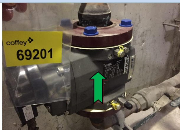
Photo 3 Interior: gas meter room, pipe work, white gasket – no asbestos detected.
