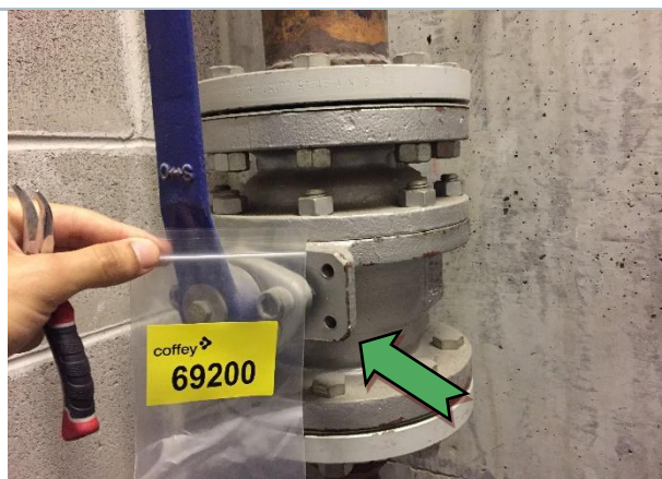
Photo 2 Interior: gas meter room, pipe work, blue gasket – no asbestos detected.
