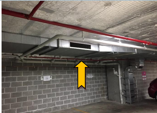
Photo 9 Interior: all levels, throughout, air conditioning ductwork – suspected SMF containing internal insulation.
