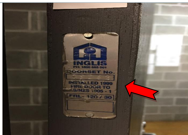
Photo 1 Interior: all levels, fire door – suspected asbestos containing fire door core.
