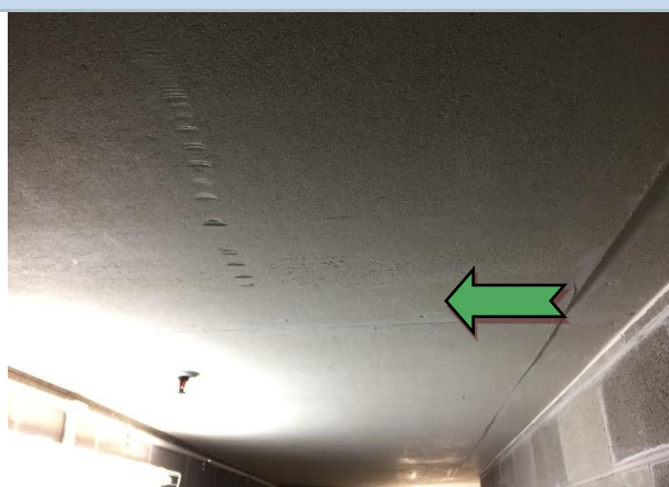
Photo 4 Interior: level 14, access corridor to cooling tower, ceiling insulation board – no asbestos detected.
