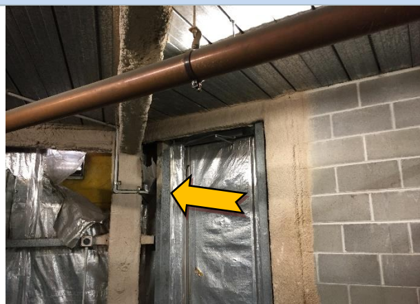
Photo 5 Interior: level 14, plant room, beams, vermiculite – no asbestos detected.
