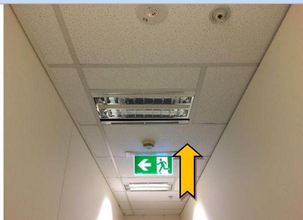
Photo 6 Interior: all levels, throughout, ceiling – suspected SMF containing compressed ceiling tiles.
