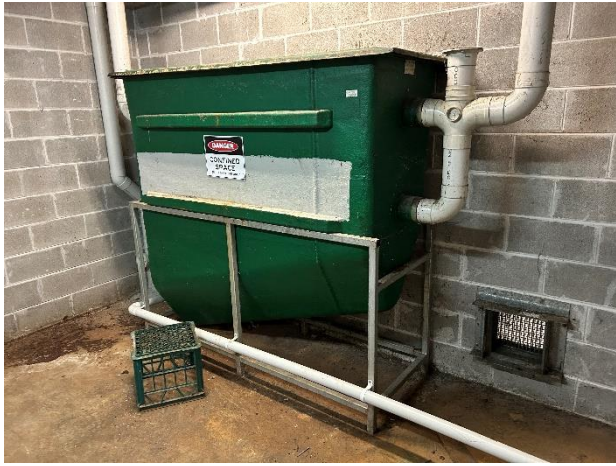
Photo 07. Level B3, Grease Arrestor Room – grease trap.
