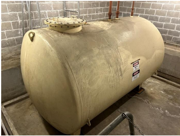
Photo 01. Diesel Tank Room – fuel tank.
