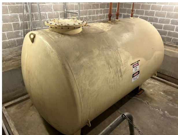
Photo 06. Diesel tank in Diesel Tank Room.
