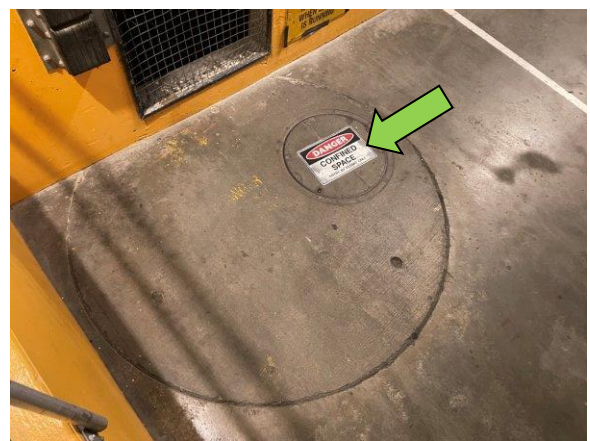
Sub soil sump pit in the Lower Ground Level Loading dock Area with appropriate confined spaces labelling
