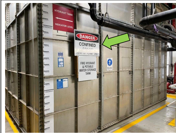
Water tanks in the Level 33 Plant Room with appropriate confined spaces labelling
