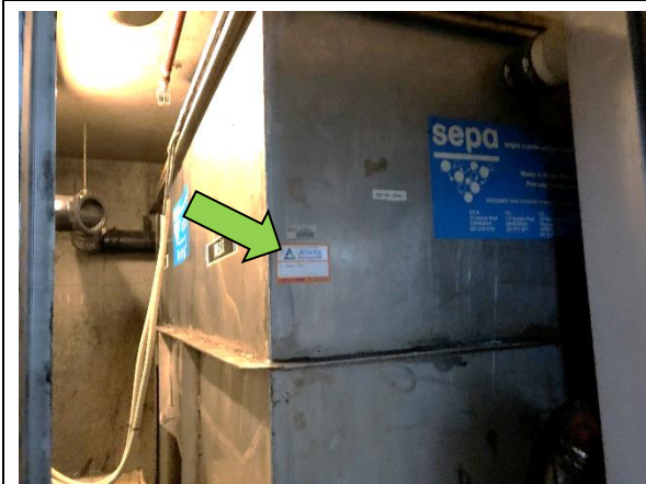
Grease Trap on Level B4 without appropriate confined spaces labelling
