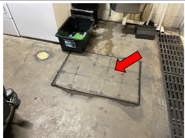
Service pit in the Cleaner's Store Room without appropriate confined spaces labelling
