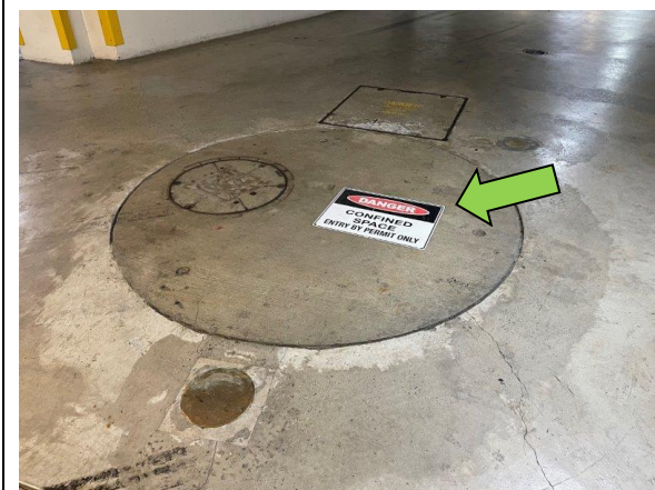
Subsoil sump pit on level in the car park with appropriate confined spaces labelling
