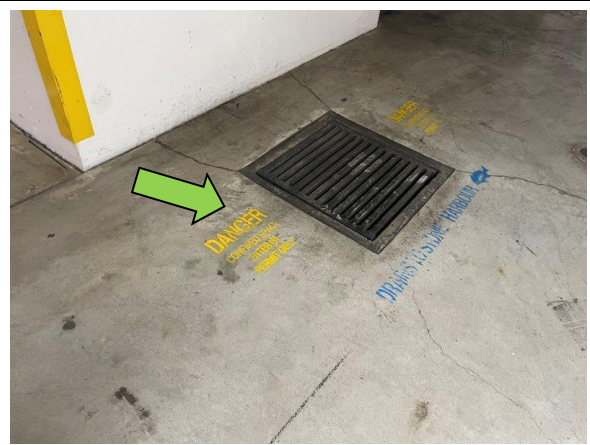
Stormwater pit on Level B5 with appropriate confined spaces labelling
