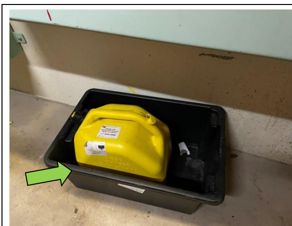
Diesel Fuel stored with appropriate bunding
