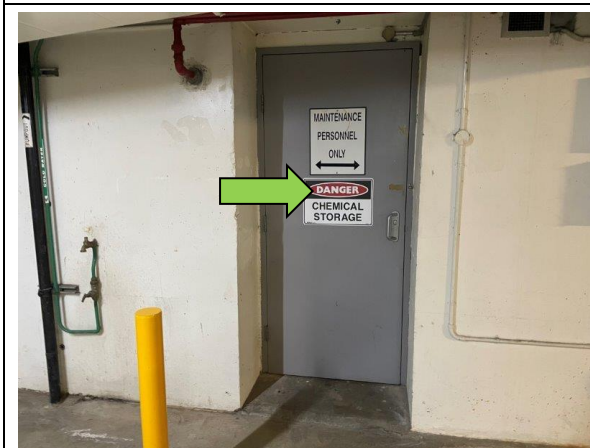
Chemical warning signage installed on the door to the Secondary Cleaners Storage Room
