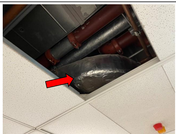
Photo 8: All Levels, Ceiling Space, Air Conditioning Duct Work – SMF insulation
