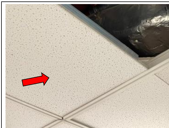
Photo 7: All Levels, Office Areas – SMF compressed ceiling tiles
