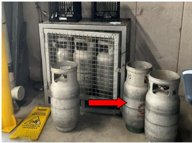
Photo 13. Inappropriately stored gas cylinders in the Greek Street Building, Dock.
