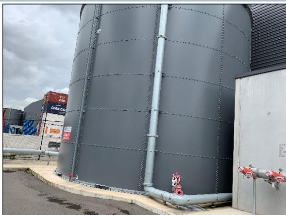
Photo 11 Exterior, ground level, north western corner of building, water storage tank (Fire Sprinkler 512kL)
