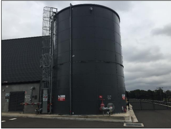
Photo 27 Exterior, ground level, north eastern corner of building, water storage tank (Sprinkler Tank 545kL)
