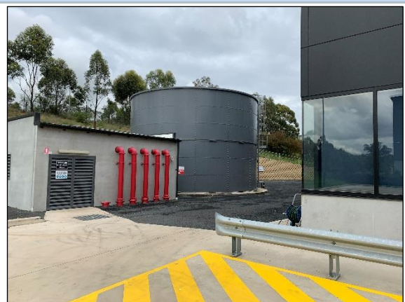
Photo 33 Exterior, ground level, southern corner of building, water storage tank (Sprinkler Tank 580kL)
