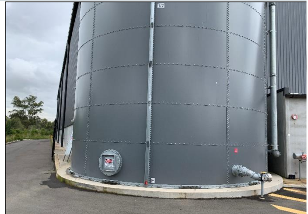
Photo 43 Exterior, ground level, south eastern corner of building, water storage tank (Sprinkler 545kL)
