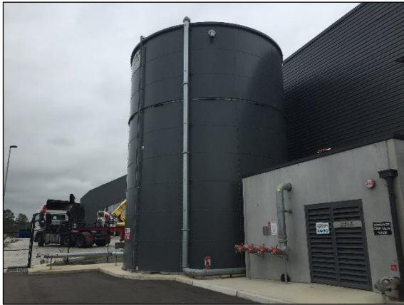
Photo 20 Exterior, ground level, south eastern corner of building, water storage tank (Sprinkler Tank 545kL)
