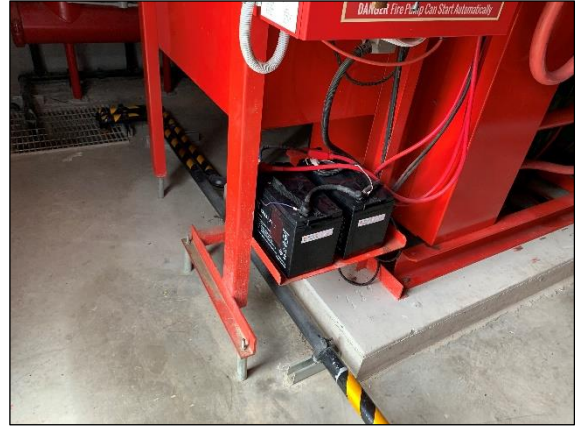
Photo 2 Battery storage within Sprinkler Pump Rooms.
