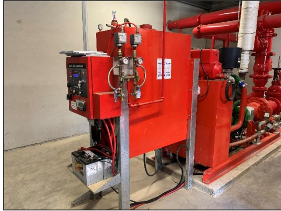
Photo 1 Diesel fuel storage within Sprinkler Pump Rooms.
