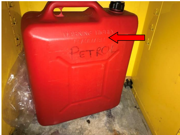
Photo 9. Level B5, Cleaners Room, Flammable Cabinet – Inadequately labelled chemical containers.
