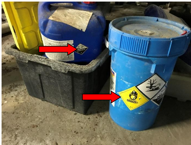
Photo 1. Level 7, Cooling Tower Plant Room – Inadequate chemical segregation.
