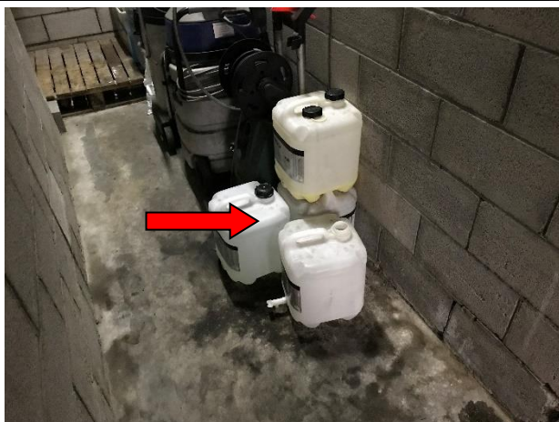
Photo 11. Level B1, Kitchen Exhaust EF36 & EF47 – No spill containment.
