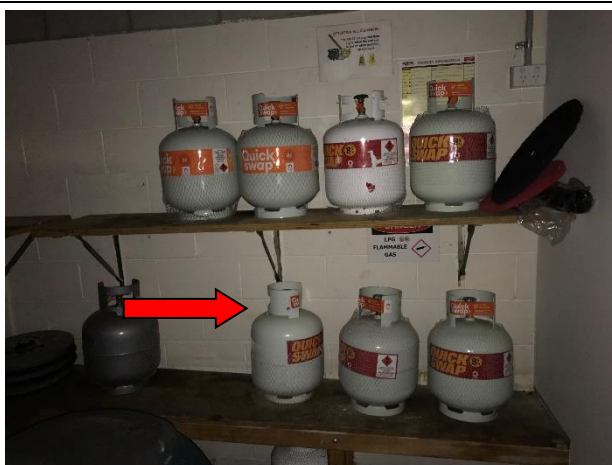
Photo 5. Level B5, Cleaners Room – Gas cylinders not appropriately stored.
