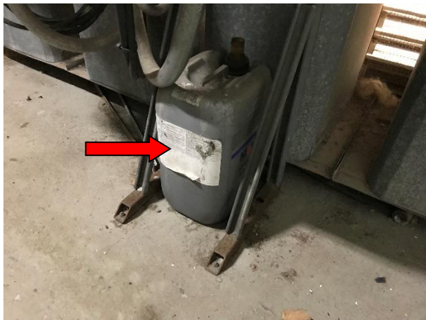
Photo 13. Level 7, Cooling Tower Plant Room – No spill containment.
