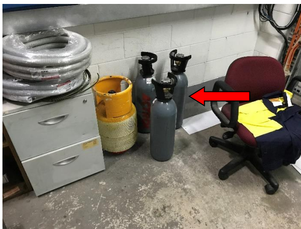
Photo 3. Level B3, Plant Room 3.10 – Gas cylinders not appropriately stored.
