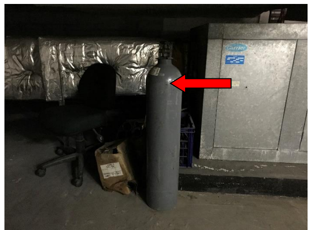
Photo 4. Level B3, Plant Room 3.10 – Gas cylinders not appropriately stored.
