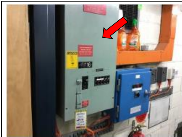
Greenwood Plaza, Level 7, Lift Motor Room – electrical backing board suspected to contain asbestos
