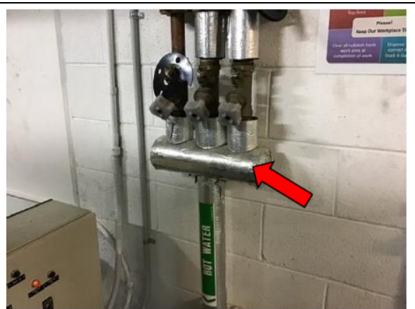
Throughout Building – SMF insulation to pipework
