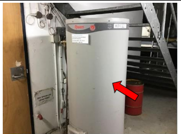
Example of SMF internal insulation in hot water heaters on site
