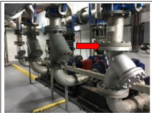
101 Miller Street, Level 8, Chiller Room – pipework gaskets throughout confirmed to contain asbestos
