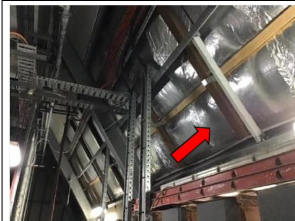
Plant Rooms – SMF insulation to ceiling (behind sarking)
