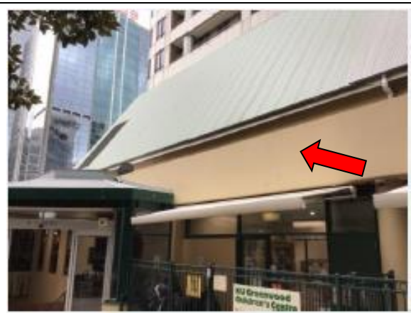
Greenwood Plaza, Roof Level – Fascia fibre cement suspected to contain asbestos
