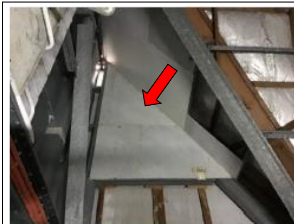
Greenwood Plaza, Level 7, Switch Room – Infill Panels fibre cement suspected to contain asbestos
