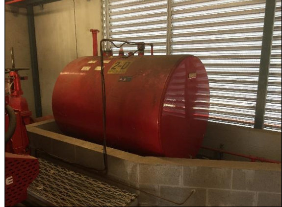
Photo 2 Diesel fuel storage within 40 Blackbird Close Sprinkler Pump Room.
