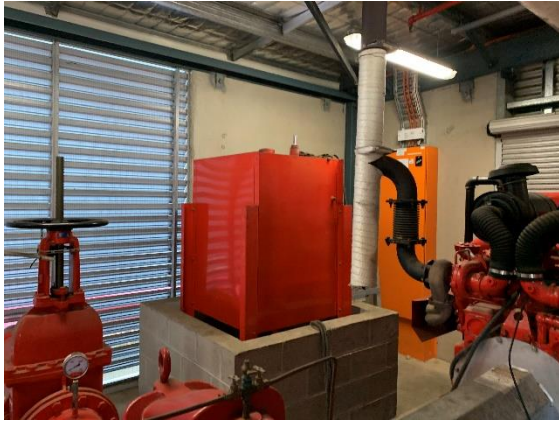
Photo 1 Diesel fuel storage within 40 Blackbird Close Sprinkler Pump Room.
