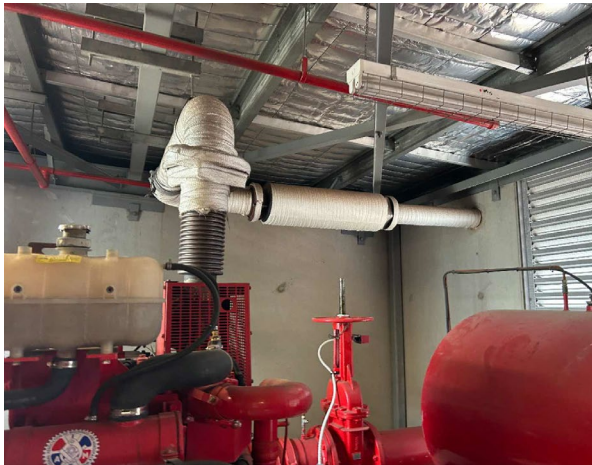
Line ID 1: Internal, GL, Northern Fire Pump Room, Pump Exhausts, Insulation Material - Suspected SMF
