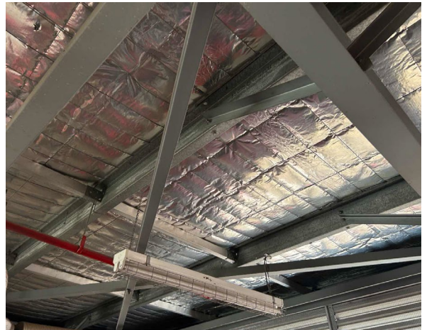
Line ID 2: Internal, GL, Northern Fire Pump Room, Underside of Ceiling, Sarking Insulation - Suspected SMF
