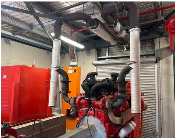
Line ID 3: Internal, GL, Southern Fire Pump Room, Pump Exhausts, Insulation Material - Suspected SMF
