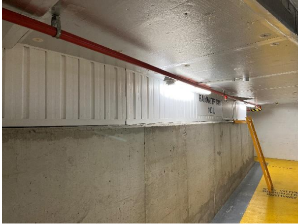
Photo 07. Mezzanine Level, Plant Room, Rainwater Tank 100kL
