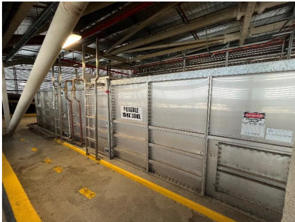
Photo 11. Level 6, Plant Room, Potable Water Tank 30kL
