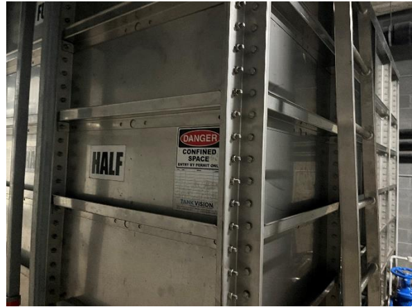
Photo 18. Lower Ground, Rainwater Tank Room, Rainwater Tank 8kL.
