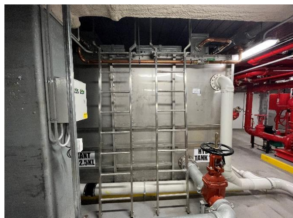
Photo 16. Lower Ground, Sprinkler Tank and Pump Room, Hydrant Water Tank 12.5kL
