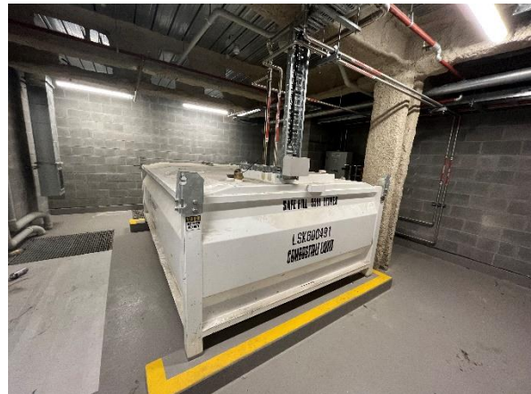
Photo 28. Bay 15 Ground Level Generator Room, diesel tank
