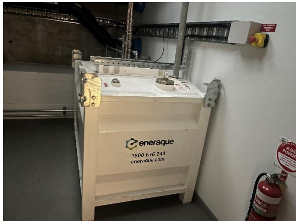
Photo 27. Bay 15, Generator Room, diesel tank
