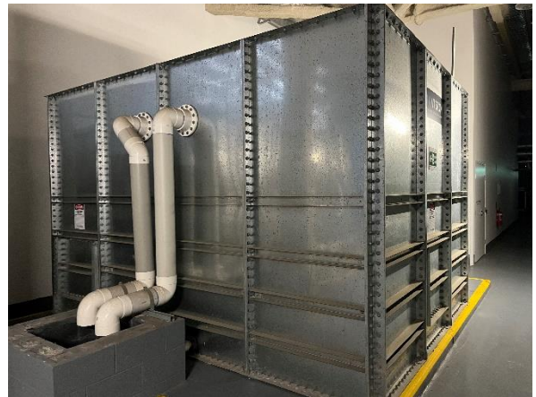
Photo 10. Level 8, Plant Room, Hydrant Water Tank 12.5kL
