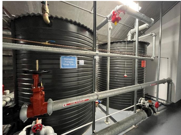
Photo 26. Fire Hydrant & Sprinkler Pump Room, Domestic Portable Water Tank x 2
