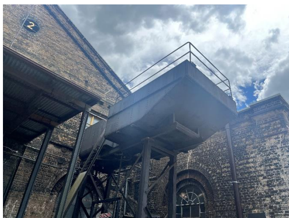
Photo 31 Exterior Bay 2, Decomissioned Water Tanks x 2
