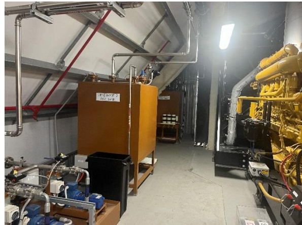
Photo 12. Level 6 Generator Plant Room, Diesel Fuel Tank x 3
