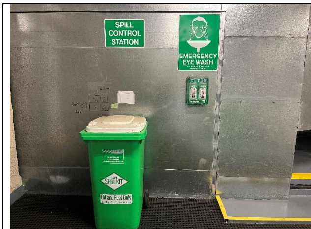
Photo 07. Spill kit and eyewash station.
