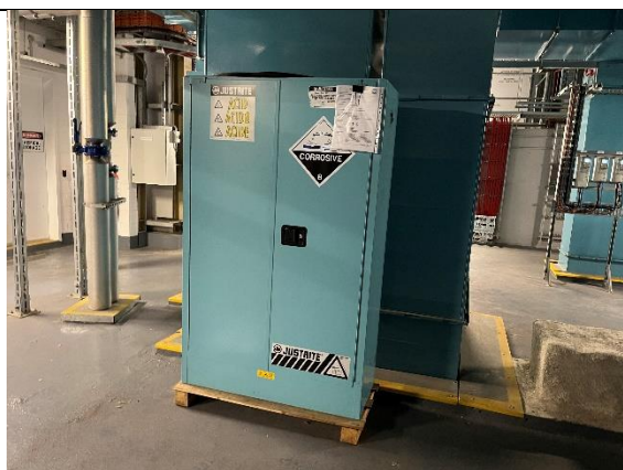
Photo 03. Level 8, Plant Room, Corrosive Cupboard, Incorrectly labelled.
