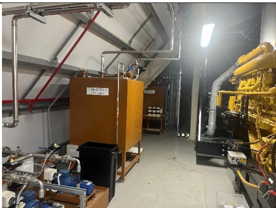
Photo 12. Level 6, generator room, diesel fuel storage.
