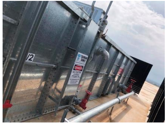
Photo 74. Confined Space 74 and 75.
