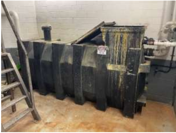
Photo 01. Level P1, Grease Arrestor Room – grease trap.
