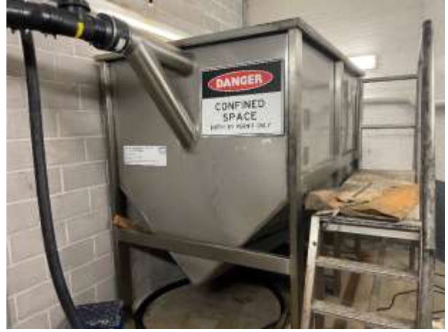
Photo 02. Level P1, Grease Arrestor Room – grease trap.
