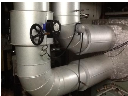
PHOTO NO.: J153823-001-PHOTO007 RESULT: SMF - PRESUMED POSITIVE BUILDING/LEVEL: MAIN BUILDING - LEVEL FIVE ROOM/LOCATION: PLANT ROOM - VARIOUS THROUGHOUT FEATURE/MATERIAL: PIPEWORK INSULATION - INSULATION MATERIAL SAMPLE NO.: -
