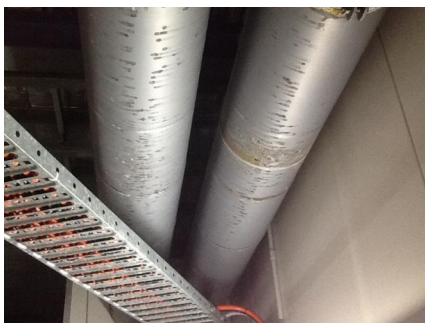
PHOTO NO.: J153823-001-PHOTO012 RESULT: SMF - PRESUMED POSITIVE BUILDING/LEVEL: MAIN BUILDING - LEVEL SIX ROOM/LOCATION: PLANT ROOM - VARIOUS THROUGHOUT FEATURE/MATERIAL: PIPEWORK INSULATION - INSULATION MATERIAL SAMPLE NO.: -
