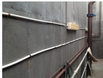
PHOTO NO.: J153823-001-PHOTO009 RESULT: SMF - PRESUMED POSITIVE BUILDING/LEVEL: MAIN BUILDING - LEVEL FIVE ROOM/LOCATION: COOLING TOWERS - THROUGHOUT FEATURE/MATERIAL: WALL - INSULATION MATERIAL SAMPLE NO.: -
