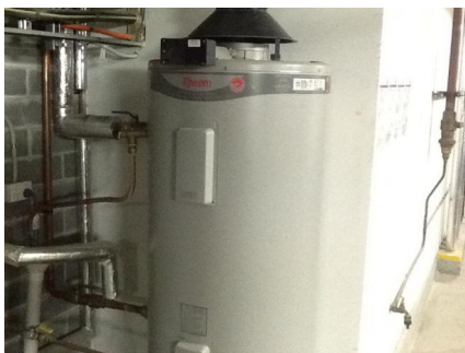
PHOTO NO.: J153823-001-PHOTO005 RESULT: SMF - PRESUMED POSITIVE BUILDING/LEVEL: MAIN BUILDING - LEVEL FIVE ROOM/LOCATION: PLANT ROOM - SOUTH FEATURE/MATERIAL: HOT WATER HEATER - INSULATION MATERIAL SAMPLE NO.: -
