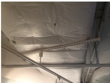
PHOTO NO.: J153823-001-PHOTO003 RESULT: SMF - PRESUMED POSITIVE BUILDING/LEVEL: MAIN BUILDING - ALL LEVELS ROOM/LOCATION: ALL ROOMS - VARIOUS THROUGHOUT FEATURE/MATERIAL: DUCTWORK INSULATION - INSULATION MATERIAL SAMPLE NO.: -
