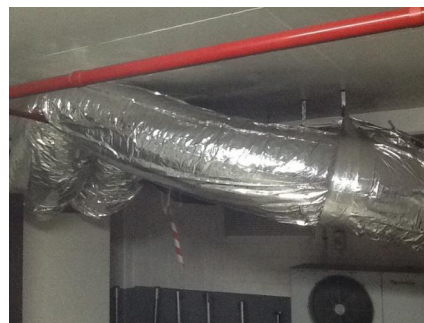
PHOTO NO.: J153823-001-PHOTO001 RESULT: SMF - PRESUMED POSITIVE BUILDING/LEVEL: MAIN BUILDING - PARKING LEVEL P1 ROOM/LOCATION: CAR PARK - SOUTHEAST FEATURE/MATERIAL: FLEXIBLE DUCTWORK INSULATION - INSULATION MATERIAL SAMPLE NO.: -
