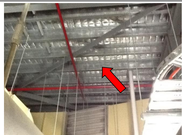
Interior, Levels 5 & 6, Plant Rooms, Roof Lining, – SMF sarking insulation material (foil-clad)
