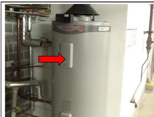
Interior, Level 5, Plant Room, Hot Water Services Tanks – SMF insulation material
