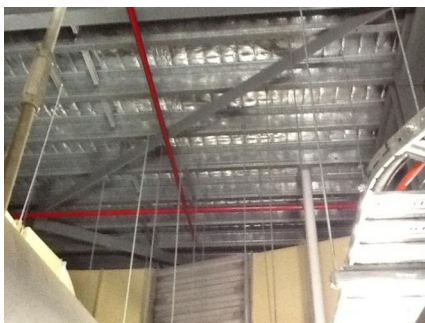
PHOTO NO.: J153823-001-PHOTO008 RESULT: SMF - PRESUMED POSITIVE BUILDING/LEVEL: MAIN BUILDING - LEVEL FIVE ROOM/LOCATION: PLANT ROOM - THROUGHOUT FEATURE/MATERIAL: ROOF LINING - SARKING INSULATION SAMPLE NO.: -
