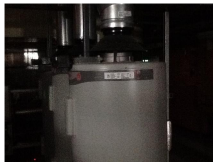
PHOTO NO.: J153823-001-PHOTO004 RESULT: SMF - PRESUMED POSITIVE BUILDING/LEVEL: MAIN BUILDING - LEVEL FIVE ROOM/LOCATION: PLANT ROOM - SOUTH FEATURE/MATERIAL: HOT WATER HEATER - INSULATION MATERIAL SAMPLE NO.: -
