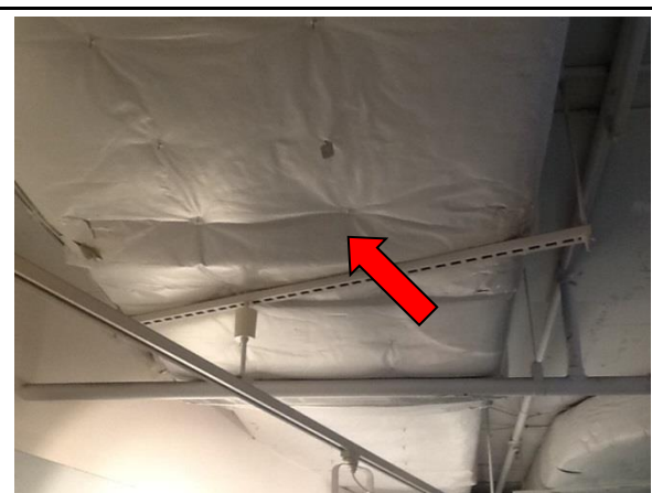
Interior, All Levels, All Rooms, Air-conditioning Ductwork – SMF insulation material (foil-clad)
