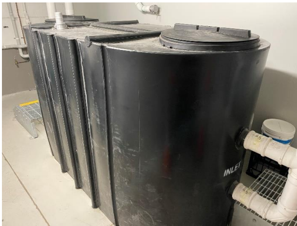
Photo 03. Level B1, Grease Trap Room – grease trap (not signposted).
